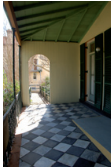
Figure 3.15 View to north-west along ground floor front veranda of residence. The roof is original but some of the cast metal work and flooring were replaced in the early 1980s. The access ramp is a later, reversible addition.
