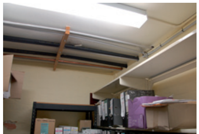
Figure 3.35 Detail of ceiling in Store (LG6), showing cabling penetrating brick wall.
