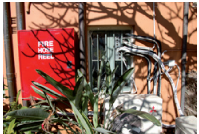
Figure 3.13 Residence north-west facade at lower ground floor, showing fire hose reel box and cabling fixed to wall and penetrating window
